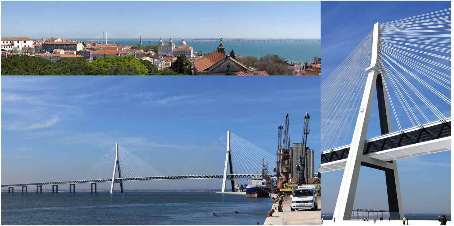
540 m main span, double level cross section 28m wide, highway traffic + Railway fixed truck
